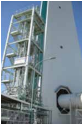
CO 2 recovery pilot plant at LNG-fired Nanko Power Station
